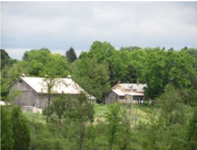
Above: Intern Farmhouse (right) and barn (left) [Photo Credit: Martina Schaefer]
